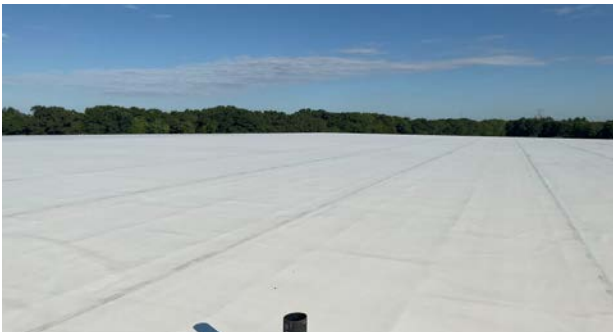
FIGURE 3: ENERGY-EFFICIENT WHITE TPO ROOFING
